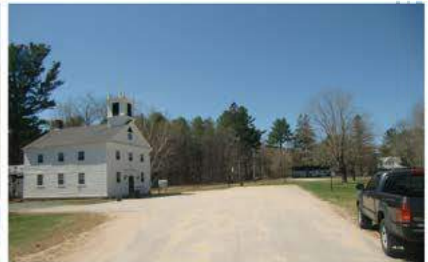
Church parking snow is pushed into the common; snow storage damage
